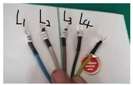
L1, L2 and L3 are phase lines; L4 is N line; the other one is PE line.
